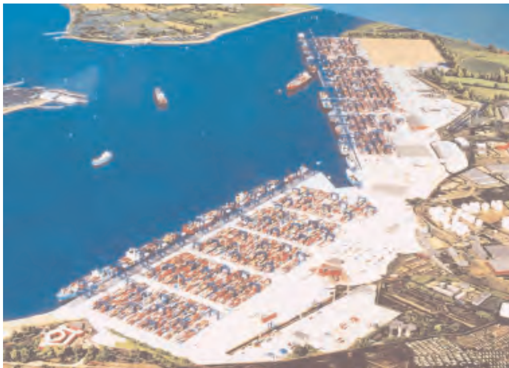
Model of the revamped Felixstowe South Quay. Landguard Point and Fort are bottom left and are to be redeveloped as a visitor attraction. The existing Trinity Quay runs away north, from what is currently the entrance to the Felixstowe Wet Dock.
